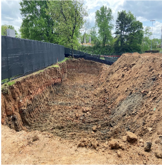
Building Pad Undercutting
