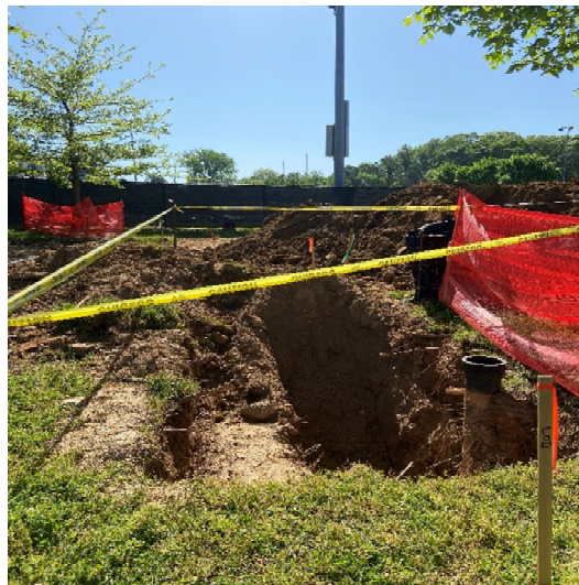
Underground Utility Trenching
