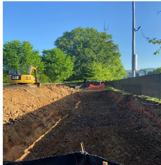
Building Pad Undercutting
